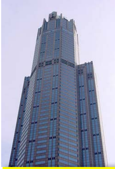
South Wacker Chicago Tower.
